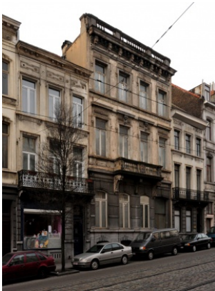
Storage place of the Mundaneum at Avenue Rogier
